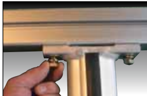
6B hand tight 16 bolts before wrenching
