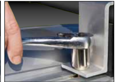
Tighten to 23 ft. lbs (31N-m).
