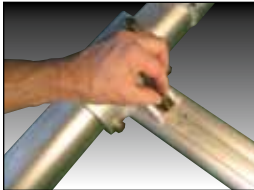
9B T-Bolts inserted
