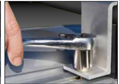
Tighten to 23 ft. lbs (31N-m).
