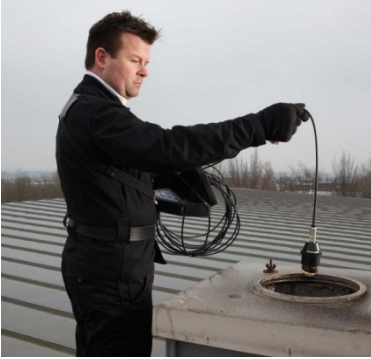
Fig. 5: Inspections using camera cable from above
