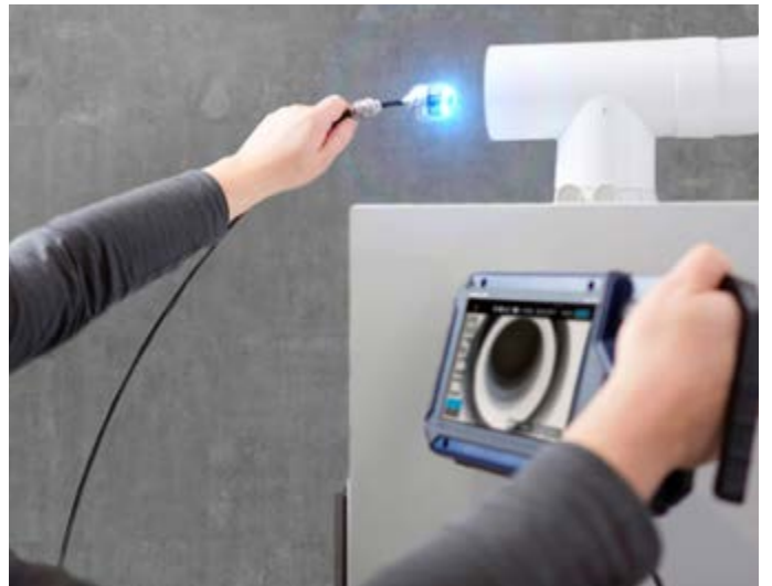
Inspection of flue gas lines from 2.2" dia. easily negotiates tight bends of 87°
