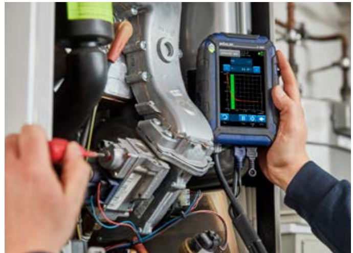
The tuning guide offers an advanced guidance to the technician to properly adjust the burner.
