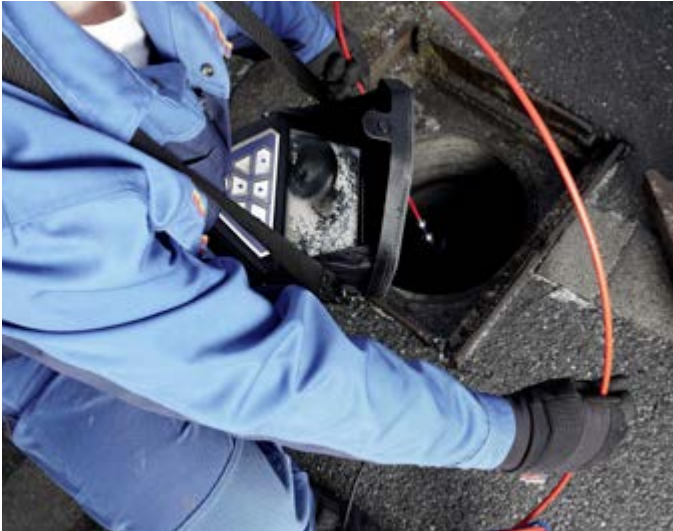
Professionally equipped with camera viper for inspecting underground pipelines
