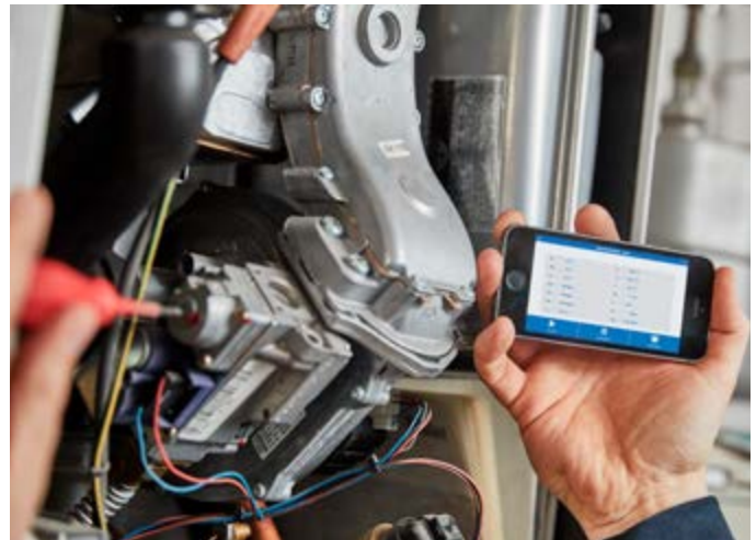
Wohler A 450 app: Displaying the measured data on a mobile device
