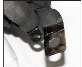
Photo 9 After Plate Removal
