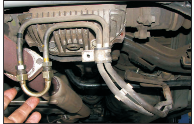
Photo 1: Hydraulic By-pass pipe
