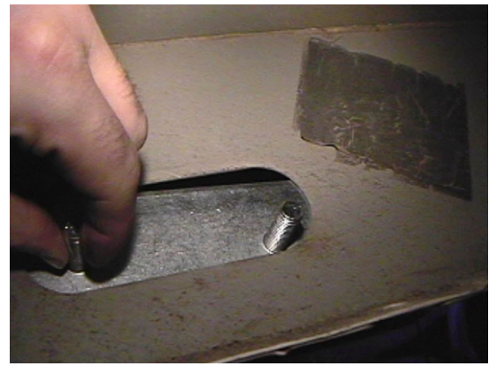
BOLT PLATE INSTALLATION FIGURE 5
