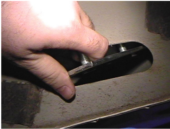
BOLT PLATE INSTALLATION FIGURE 5
