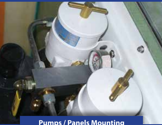
Pumps / Panels Mounting
