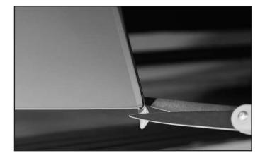
Trimming the excess material may be required depending on starting point chosen. Use a squeegee or your hand to set any remaining film into place.
