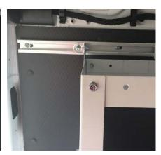
**STEP 16.** Make sure all shelves are aligned and make sure all bolts and nuts are properly torqued to spec. use 76 in-lbs for 1/4-20 hardware and 13 ft-lbs for 5/16-18 hardware.
