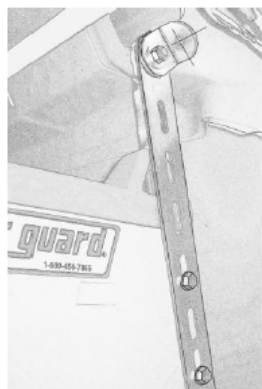
Attach Mounting Strap to end panel with 2 sets of \frac{1}{4} -20 hardware
