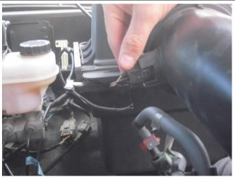
1. Disconnect the harness from the air temperature sensor on back side of factory air duct.
