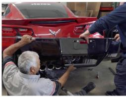
Remove the C7 rear bumper fascia. This will facilitate the installation process.
