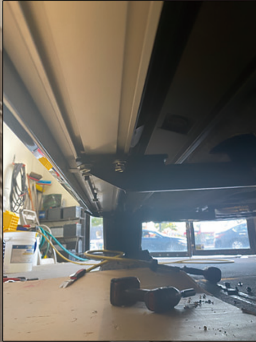
12. Pedal fixed installation completed
