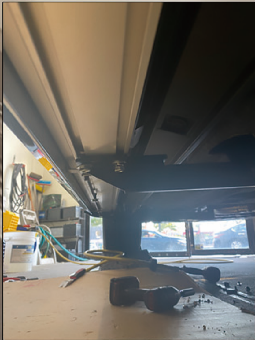
12. Pedal fixed installation completed
