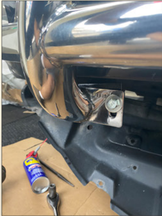
10. Bracket installation completed
