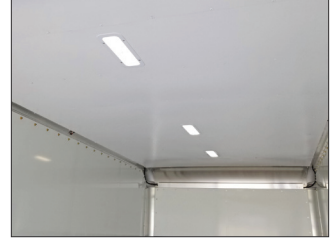
Lined and Insulated Roof
