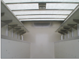
Translucent Fiberglass Roof
