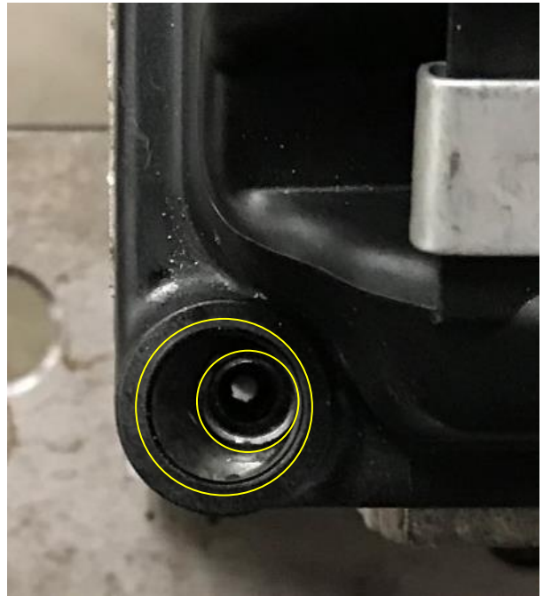
Figure 2d: Valve cover without bolt or sleeve. Housing must be forcibly deformed by installer to align fastener holes.
