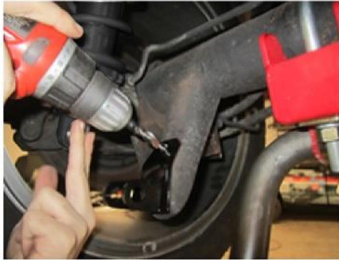
Figure 3 – Drilling for 3/8” Reinforcement
