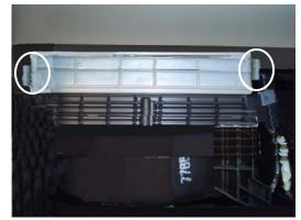
3. Push on the 2 retaining tabs to release the filter access door. Slide out the filter frame, replace old filter with <u>new TYC filter</u>, making sure Air Flow arrow is pointing down.
