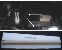
3. Grab the handle and slide out the first filter frame.
