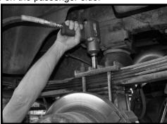
8. Locate the new rear traction bar brackets. Working on the driver side, install the new bracket between the u-bolts and the axle. Torque the u-bolts to 125 ft lbs. Repeat procedure on the passenger side.
