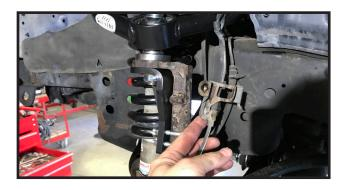
24. At this time, using a grease gun, apply grease to the 4 grease fittings located at each upper control arm eyelet. We recommend greasing until you start to see greas squeeze out of the bushings.
