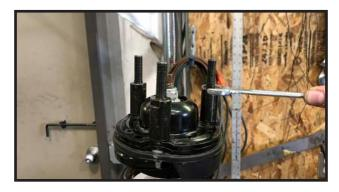
11. Locate the strut spacers part # M09151-BK-01. Slide spacer over the stud extenders, so its seated flat on the top hat.
