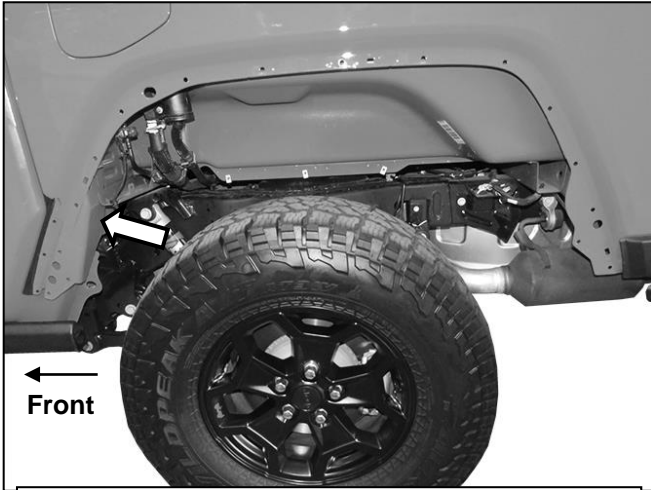
(Fig 3) Drill 25/64" hole in body panel at front location (arrow) NOTE: The mounting location cannot be accessed from between body panels
