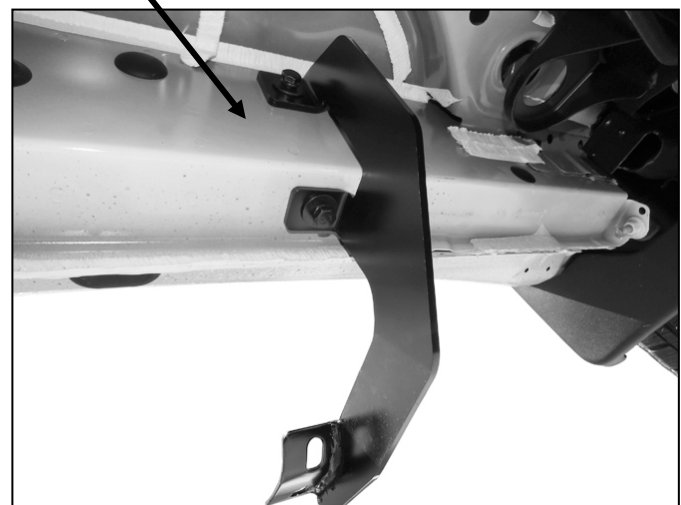
(Fig 4) Driver/left front Bracket installed
