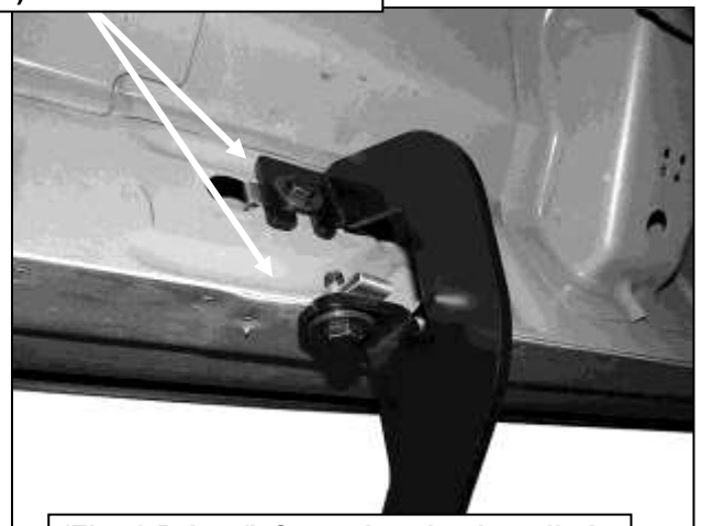
(Fig 7) Driver/left rear bracket installed
