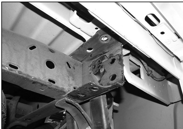
(Fig 6) End of frame once factory bumper is removed. Passenger side w-o receiver hitch pictured
