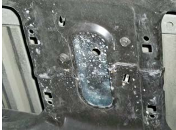
(Fig. 3) Cross member in 08-14 Ford vehicles showing STAFS top mounting plate installed.
