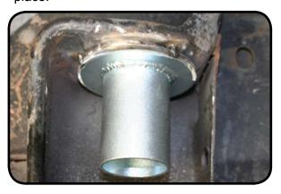
Once the bracket is in its final location, finish welding it into place. Paint all of the welding areas.
