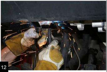
Remove any paint that has been damaged by heat and clean all welded surfaces with a wire brush. Prime and paint all welded or raw metal surfaces.
