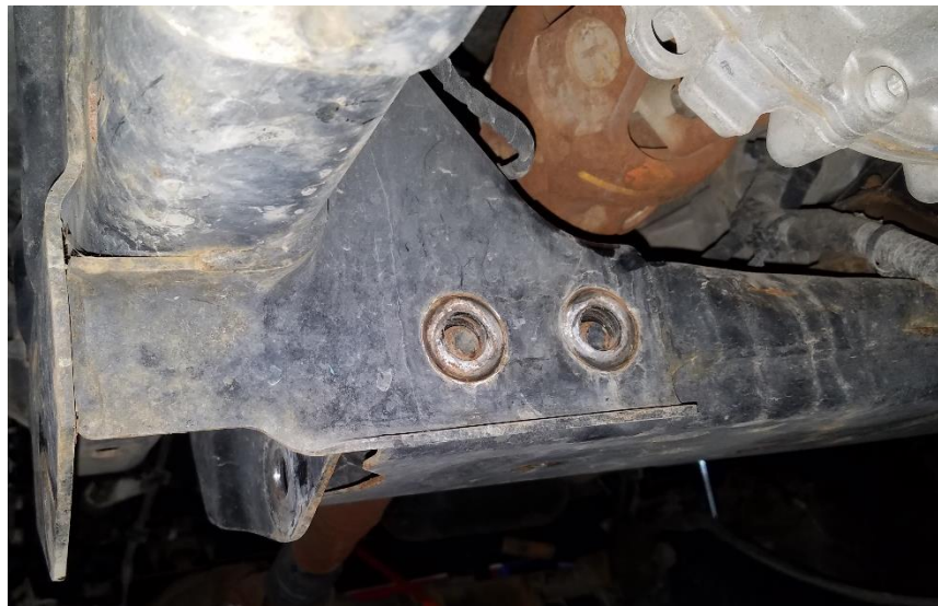
Figure 2. Transmission Cross Member Bolts Reversed
