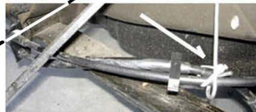
ensure cables are clear of installation
