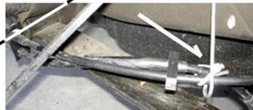
ensure cables are clear of installation
