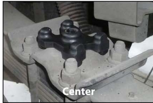
PSP7 mounted on factory spring plate
