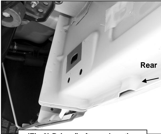
(Fig 9) Driver/Left rear location
