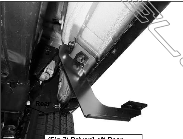
(Fig 7) Driver/Left Rear Mounting Bracket installed
