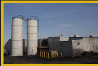
★ Plastic molding pellet silos provide ample raw material to meet any change in demand of molded product
