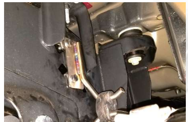
Detail 9: Frame hanger and grommet installed.
