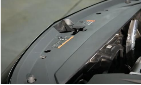
23. Reinstall radiator shroud.
