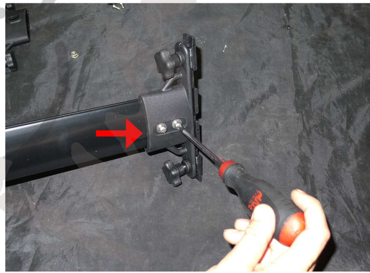
8. Secure the right side support with the (2) phillips screws
