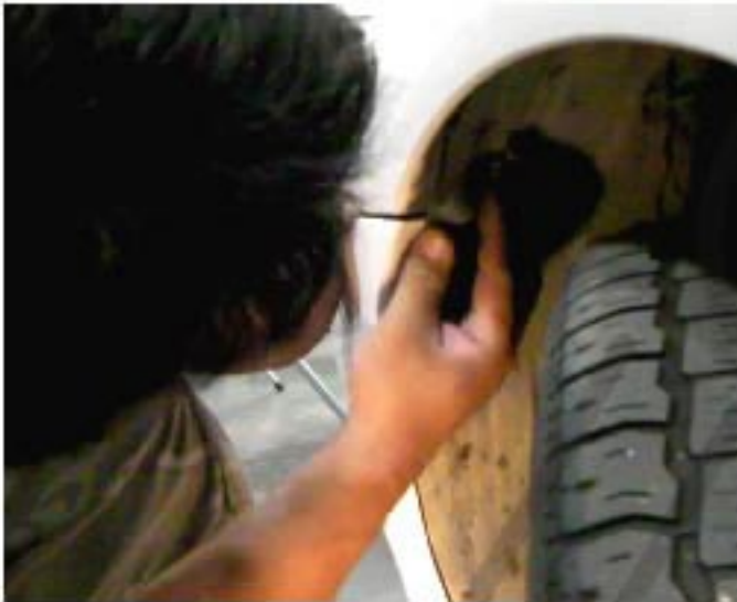
19. Install one screw inside wheel well please repeat picture order from 1 to 19 for opposite side
