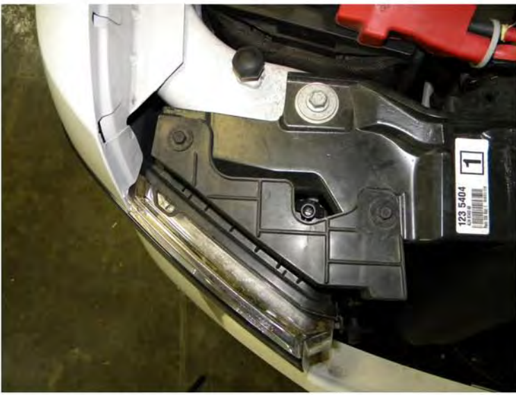
5. (2) 10mm bolts location
