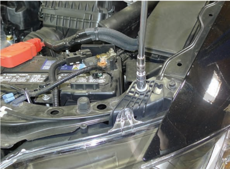
25. Tighten the 10mm bolt
