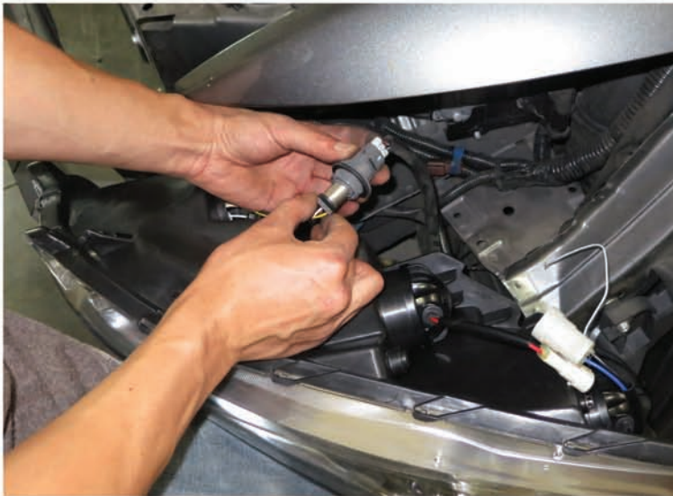
19. Connect the wire harness to the turn signal light socket Please see the " L. E. D. tail lights installation instructions" If your tail lights don't have L. E. D. You can skip the installation instructions.
