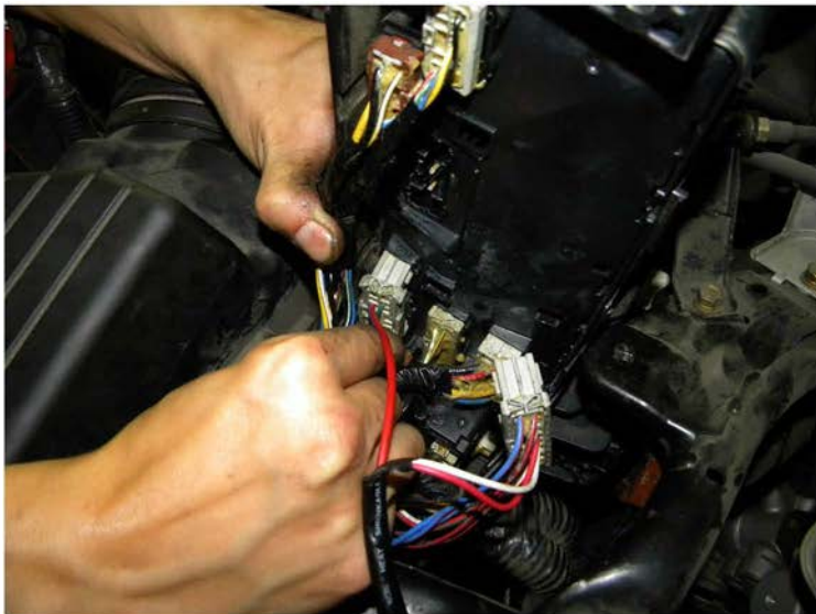
29. Reattach the connectors to the fusebox
