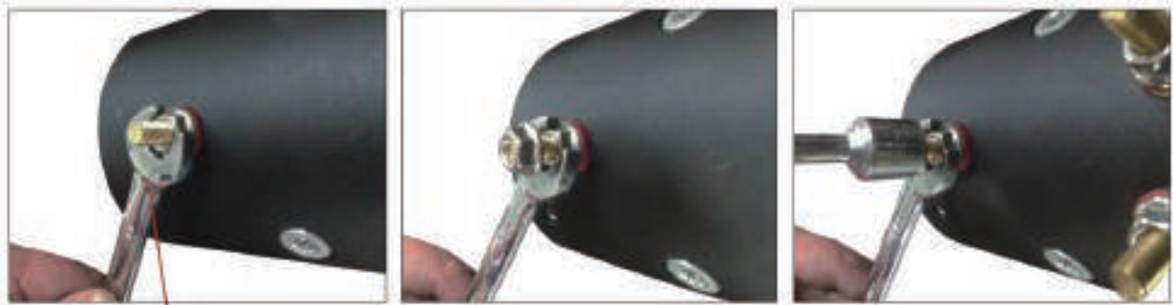
Use wrench to prevent movement of bottom lock nut when installing power cables.
