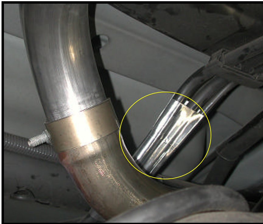
Photo 11: Fuel Lines Wrapped with Heat Tape
