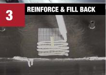
Mask front side of repair to prevent repair material from flowing through. Apply Plastic Repair Contouring Tape (mesh only) to back side. Apply Dual-Mix™ Multi-Plastic Repair Material or Dual-Mix Problem Plastic Repair Material and cover mesh tape. Spread material firmly. Allow to set.
