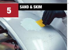
Sand with P80 grit. Finish with P180 grit. If needed, use a skim coat of **Bumper Bite™ Flexible Glaze**, then sand with P180 − P320 grit.
