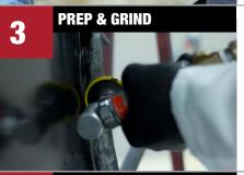
Clean with SEM Solve or XXX Universal **Surface Cleaner.** Grind mating flanges with a P36 grit grinding disc at low speed for aggressive grind mark. Remove any adhesive or protective coatings.
