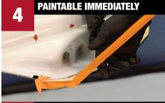
Remove masking tape immediately after clean up. Paint immediately with **Factory Pack**<sup>TM</sup> or most solvent-based coatings.
